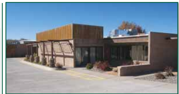
Montrose • 675 Industrial Blvd.
